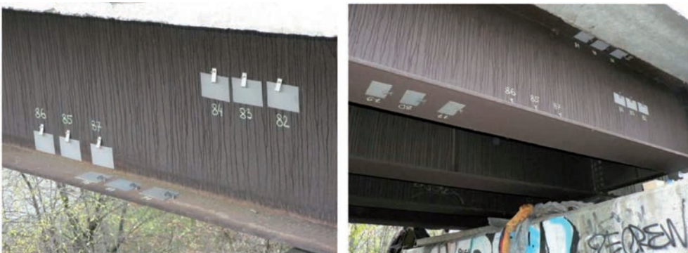
Figure 3: The installation of corrosion specimens on the railway bridge in Prague - Motol
