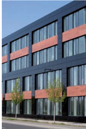
II. 6 Black cladding of glass CIGS modules – Sulfrucell building in Berlin Adlershof [13]
