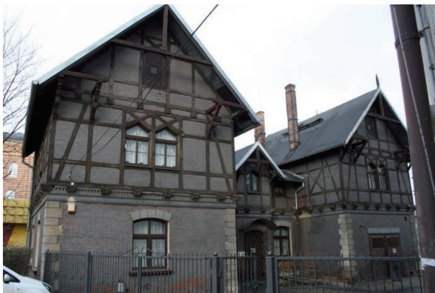
II.8. The Prussian wall in the building of the State Music School in Gliwice, A. Szymanowska-Gwiżdż 2015
