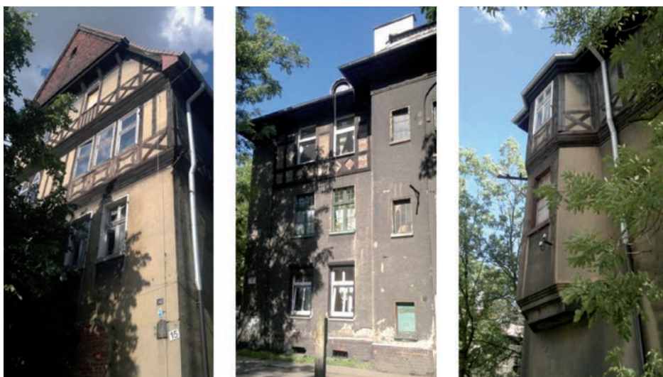
II.2-4. Wooden details of the Prussian wall in the residential buildings in Zandka settlement in Zabrze, A. Szymanowska-Gwiżdż, 2016
