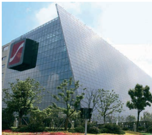
Il. 5 Research and Development Centre, Wuxi Suntech Power, Wuxi. BPV glass façade is created by 2552 semi-transparent photovoltaic panels with a total area of 20 000 m 2 . Photo Suntech [5]
