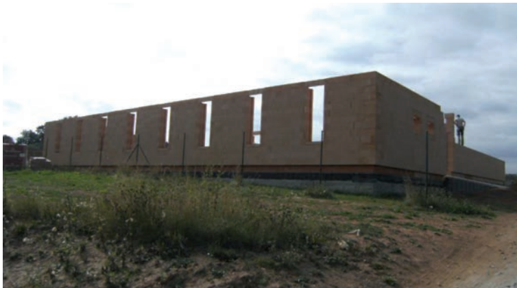
Figure. 8 Construction in September 2016. Photo: M. Nedvěď
