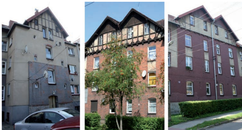
II.5-7. View of the residential buildings in the railway settlement in Pyskowiec, an originally non-usable attic made of the Prussian wall, A. Szymanowska-Gwiżdż, 2014
