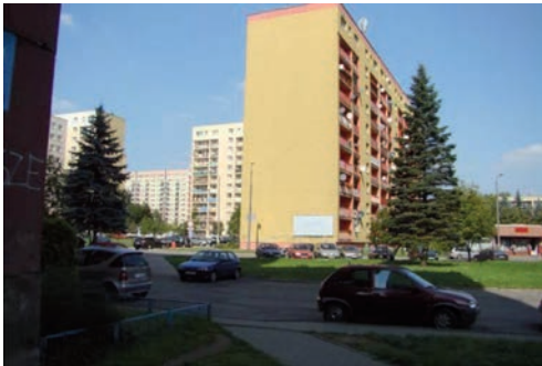
II.14. Peak wall of the building.
