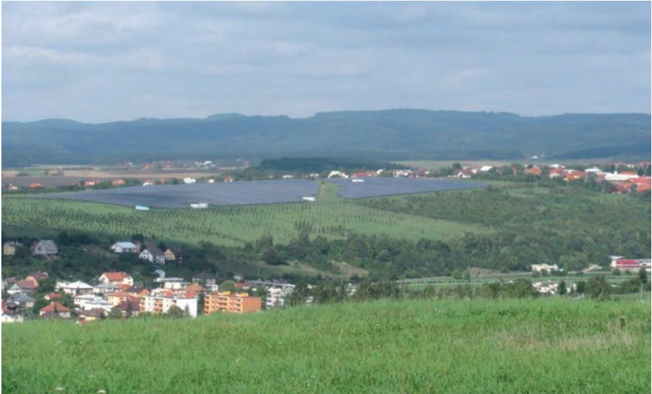
Figure.1., Plant for using solar energy near Slusovice – Czech Republic, Vojvodikova, 2015
