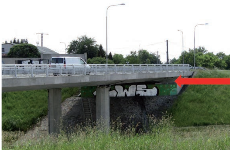
Figure 10: The concrete bridge structure under the street Ostravská (located above the bridge D1)
