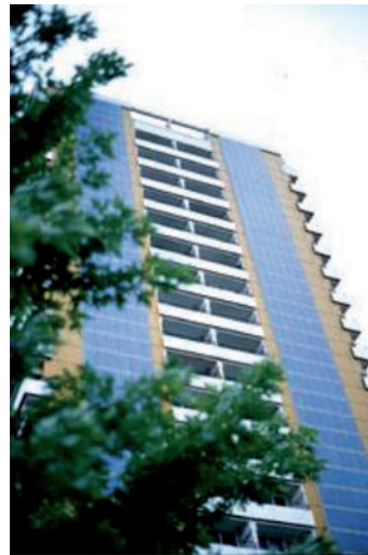
II.9. View of the façade. Source: [9].
