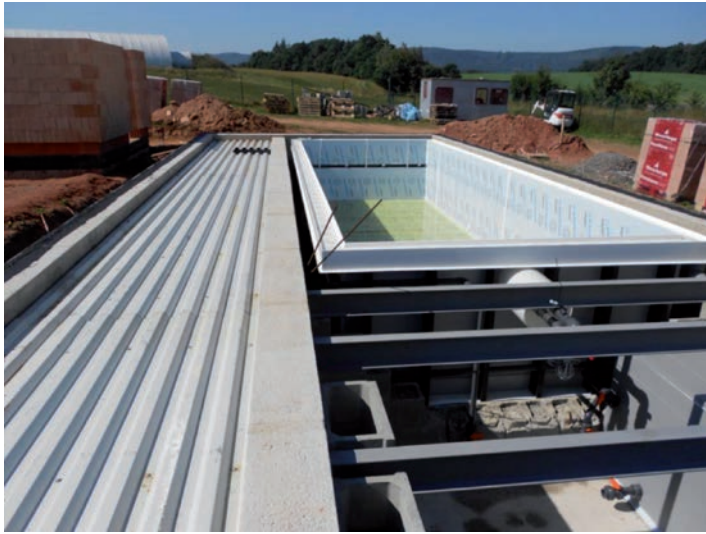
Figure. 7 Construction in August 2016. Photo: M. Nedvěď
