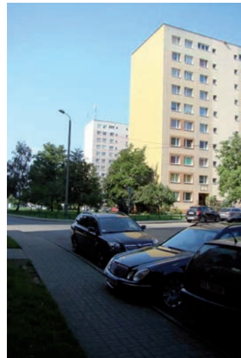
II.15. View of the buildings of the settlement at Felińskiego Street in Miechów. Source: photo by Joanna Biedrońska August 2016.
