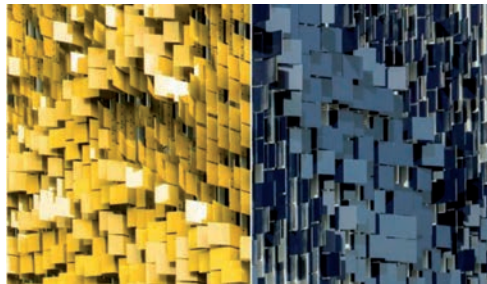
Il. 11 Close-up on the metal panels on the façade of the car park of Eskenazi hospital in Indianapolis [17]
