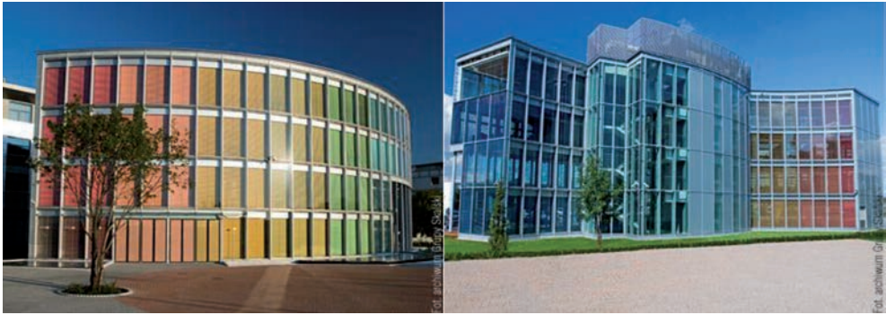
Il. 4 Coloured shutters are decorative and protect against sunlight due to the intelligent control, photo the archive of Grupa Skalska [10]
